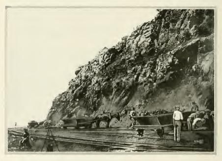
An ironstone quarry in the Iron Knob Mountain. Both the Iron Knob and the Iron Monarch mines are owned by the Broken Hill Company and the ore mined there is shipped by private railway to False Bay, then by steamer to Newcastle, where it is used in the Broken Hill Company's great steel plant.
