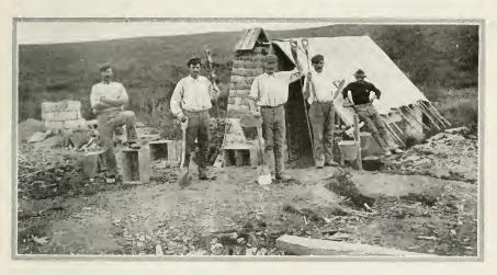
The best kauri gum is found ten or twelve feet below the surface of the ground, where ancient kauri forests are buried. The presence of the hidden treasure is determined by "spearing the ground." Long spearlike iron rods, such as are shown in the hands of the men in the photograph, are used to probe thru the soil and pipestone clay. Having located the gum in this manner, the diggers resort to pick and shovel. The picture shows a typical kauri gum diggers' camp.
