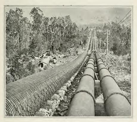
The pipes which carry the water from the Great Lake of Tasmania to the power house of the island's greatest hydro-electric development. The pipe on the left is of wood and was built during the war when steel could not be obtained. It is two miles long and forty-nine inches in diameter and is said to be the largest wooden pipe carrying water to a 400-foot head in the world. It is made of eucalyptus staves, held together by wire.
