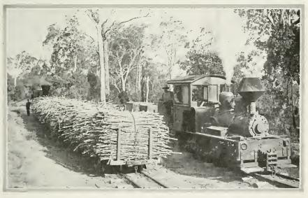
The State Railways' report asserts that Queensland owns thirty miles of "narrow gauge" railway. Elsewhere in the world a railroad three feet six inches in gauge is standard narrow gauge. That is the widest gauge in Queensland and the narrow gauge lines are two feet wide. For the most part, they operate in the sugar cane districts, where diminutive engines pull low trucks loaded with cane from the fields to the mills.
