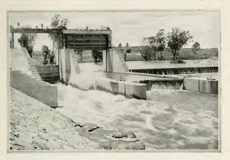
Irrigation is reclaiming thousands of barren acres in Australia. The Victorian farmer has been a leader and pioneer in irrigation. The picture shows a flood gate in one of the more extensive irrigation systems operating in Victoria.
