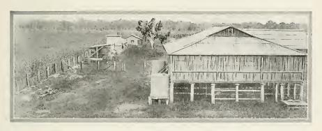
Settlers in the tropical Northern Territory of Australia, the only district which has not attained to statehood, have two pests to fight—ants and flying insects—and foil them by building their houses on stilts and inserting a tin between the piles and the floor of the house. Insects are kept out and the houses kept cool by sides of reeds fastened to light wood frames. Roofs, as elsewhere in Australasia, are of corrugated iron. The same material is used for the ever-present water tank.
