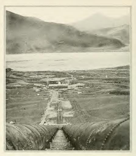
New Zealand is very rich in potential water power. In time her hydro-electric developments will make her independent of fuel. The picture shows the power house of the Lake Coleridge hydro-electric plant and the great pipes which carry the waters down the mountain from Lake Coleridge.
