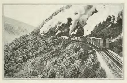
Pulling up what is said to be the steepest railroad grade in the world, over the Rimutaka Mountains, where for three miles the tracks drop one foot in every fifteen. Special locomotives, with steel shoes to grip a center rail as a brake, are used to handle trains on these grades. Terrific winds sweep these mountains, and windbreaks are built to protect the trains. On two occasions trains have been blown from the tracks.
