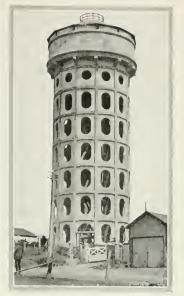
In Hamilton, one of the prosperous secondary cities of North Island, they have broken away from the conventional "stand pipe" as a source of water pressure. The steel and concrete skeleton of this water tower is encased in a concrete shell which gives the impression of a mediaeval tower.
