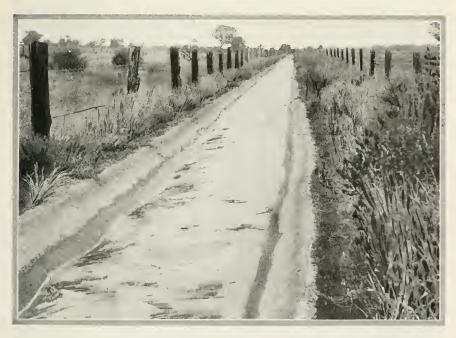
Hundreds of miles of these concrete-lined channels carry the waters of the Murray, longest river in Australia, into the arid lands which otherwise would not be productive because of the scant rainfall. This channel is part of the extensive irrigation system in the Berri district, noted for its splendid fruit. The state, which is back of all irrigation projects, builds dams and reservoirs and digs channels, and charges settlers for water equaling twenty-four inches of rain a year.
