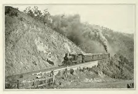
Australia has railroads in assorted sizes—wide, standard, and narrow gauge. This road up Mt. Morgan is a standard gauge, but it has three rails. The middle rail is cogged and it is used both for tractive power, as the engines toil up the steep grades, and for braking, when the train is coming down the mountain.
