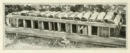
This treadmill, in the days when Tasmania was a penal colony, was used to turn a gristmill. It was operated by convicts and the heavy cleats are deeply grooved, having been worn down by the feet of the men who walked many weary miles on the machine without advancing.
