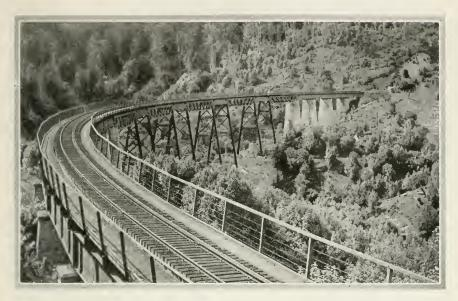
Viaducts of steel and concrete have replaced the wooden bridges on the main lines of the government railways. There are scores of them, because railroad building in New Zealand is a difficult task on account of the mountains and streams. Tunnels are frequent. One of them, now under construction on the South Island, will be five miles long.
